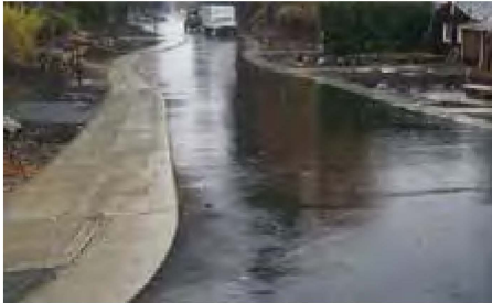
Invisible curbs along the street edge allow runoff to move into bioretention swales.
