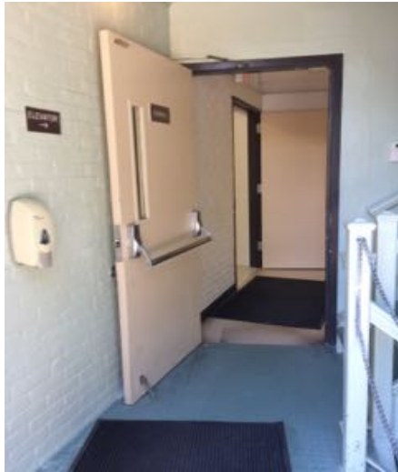
First floor vestibule clearances non-compliant & no power door opener
