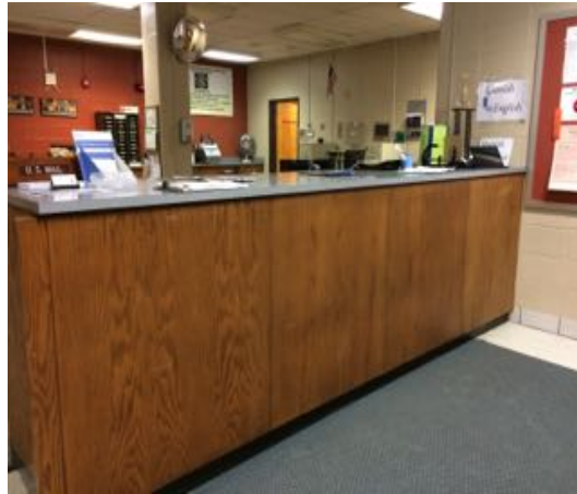
Reception/office counter has no lowered counter section
